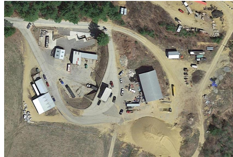
Aerial view of Transfer Station on Dump Road
