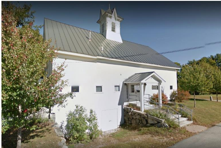
Loudon Community Building on South Village Road
