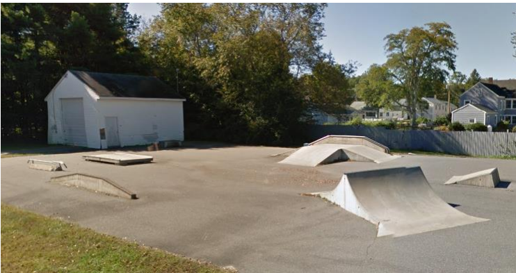
Recreational Fields and Skate Park on South Village Road & Recreation Drive
