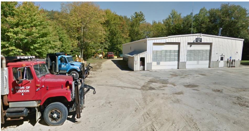
Loudon Highway Garage on Clough Hill Road
