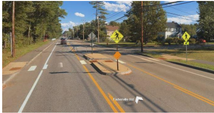
REFUGE ISLAND ON ROUTE 3 IN PENACOOK
