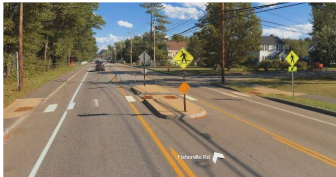
REFUGE ISLAND ON ROUTE 3 IN PENACOOK
