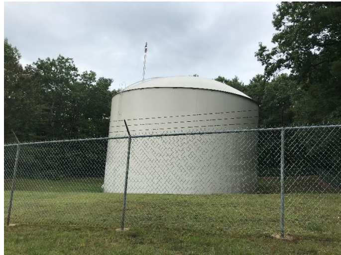
WATER STORAGE TANK ON BRICKETT HILL ROAD
