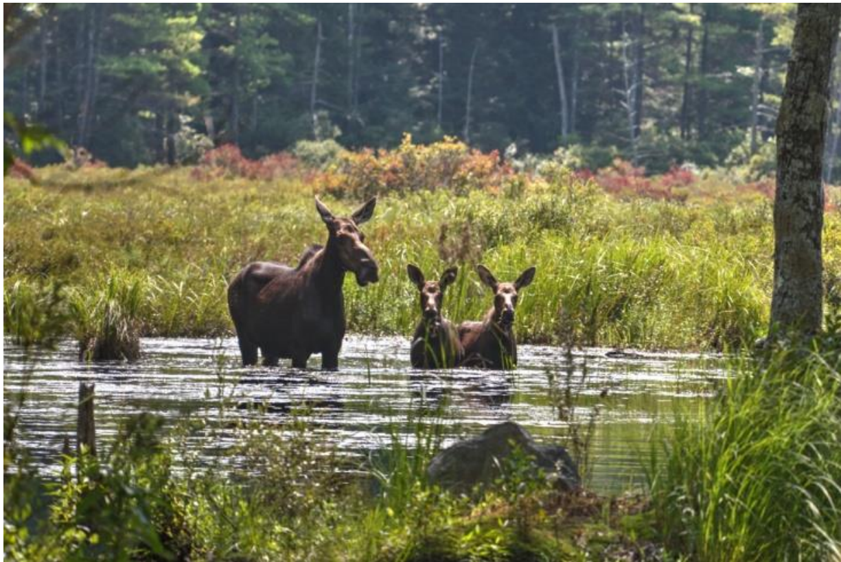
Moose viewed along Forest Street. These moose are enjoying the wetland that has been preserved by the addition of a beaver exclusion device. This device maintains a water level that works for both the beavers and the road/culvert. Photo Credit: Bill Duffy
